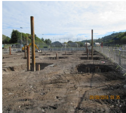
19a Piling installation
