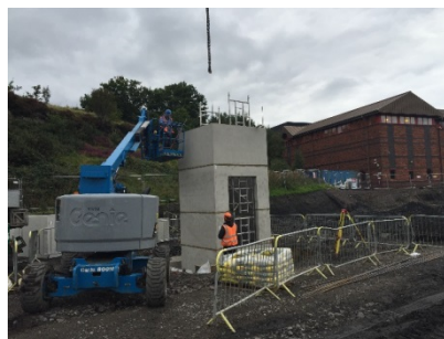
21 First lift shaft being constructed
