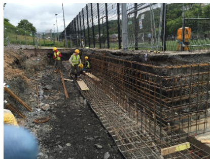
13 Construction of new retaining wall to 3G pitch
