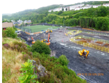
11 Preparation of concrete foundations
