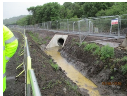
8b. Realigned culvert
