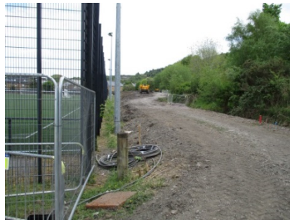
5 Core Path upgrade works adjacent to existing 3G pitch
