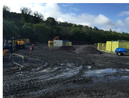
2 Preparation of site compound area
