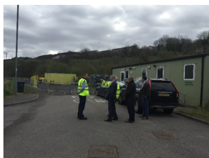
1 Existing units refurbished and used as site offices
