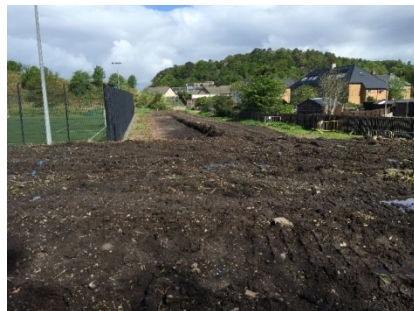
15 Excavation works for the new long/triple jump run up and sand pit
