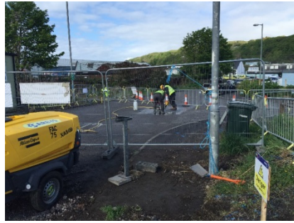
9 Drainage connection works at McCall Terrace
