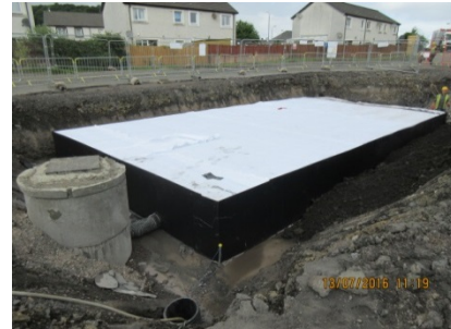
18 Attenuation tank installed
