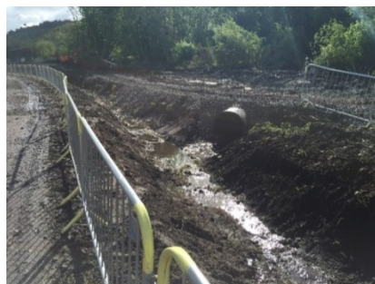
8a Culvert realignment works
