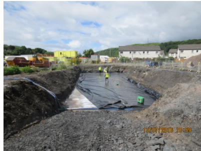
17 Preparation of site for attenuation tank
