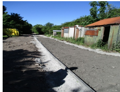
6 Core Path upgrade works at Dalintart
