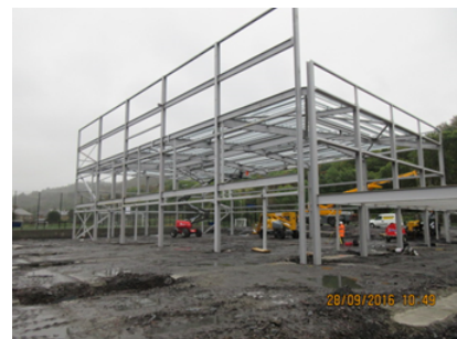
22 First sections of steelwork being erected
