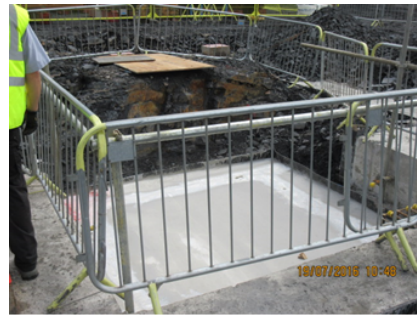
12 Concrete foundations for one of the lift shafts
